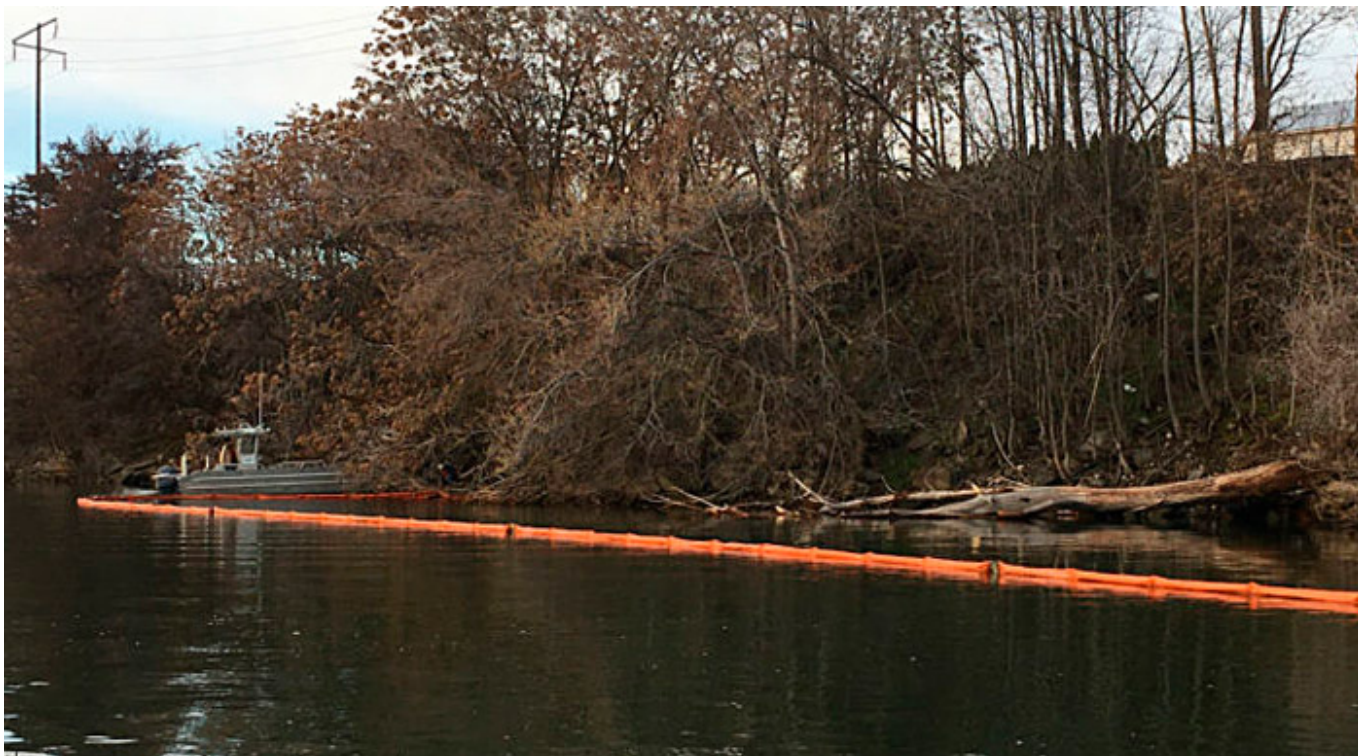
Figure 2: Placement of booms to prevent an oil sheen from spreading in the Columbia River.
